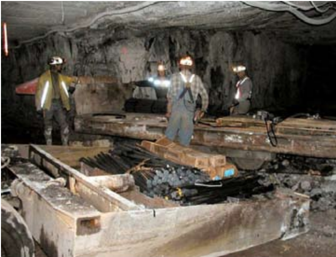
Off-loading roof bolt supplies from a trailer to a scoop underground.
