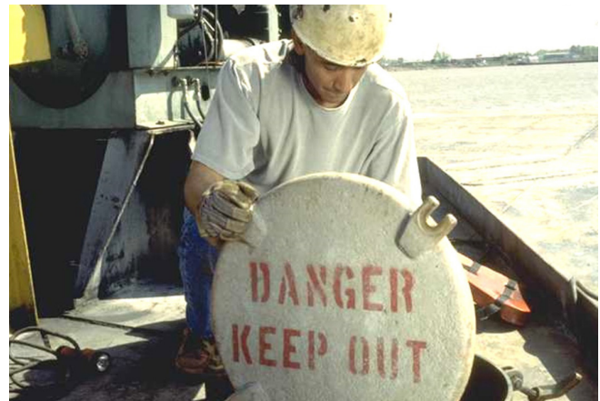
Confined space entry occurs whenever you break the plane of the opening to the space.
