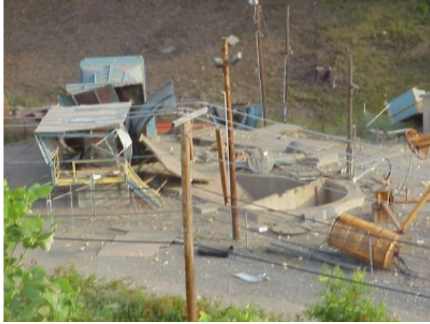
Figure 2. Damaged Surface Facilities
