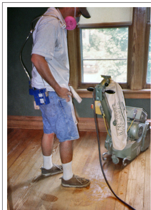
FIGURE 4.1 Sanding wooden floors can generate significant amounts of dust.
