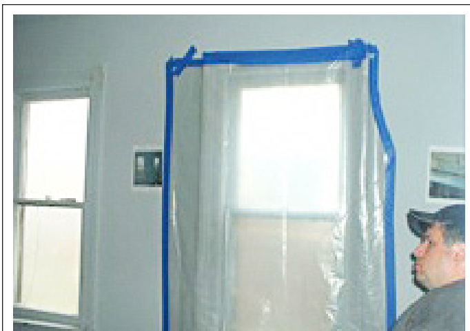
FIGURE 12.2 Protecting the interior of a unit for exterior window abatement.
