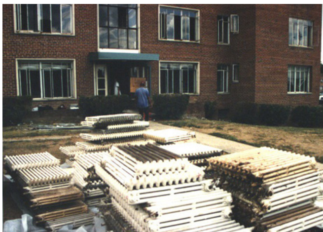
FIGURE 10.2 Radiators and trim are examples of intact architectural components that are low-level lead waste.
