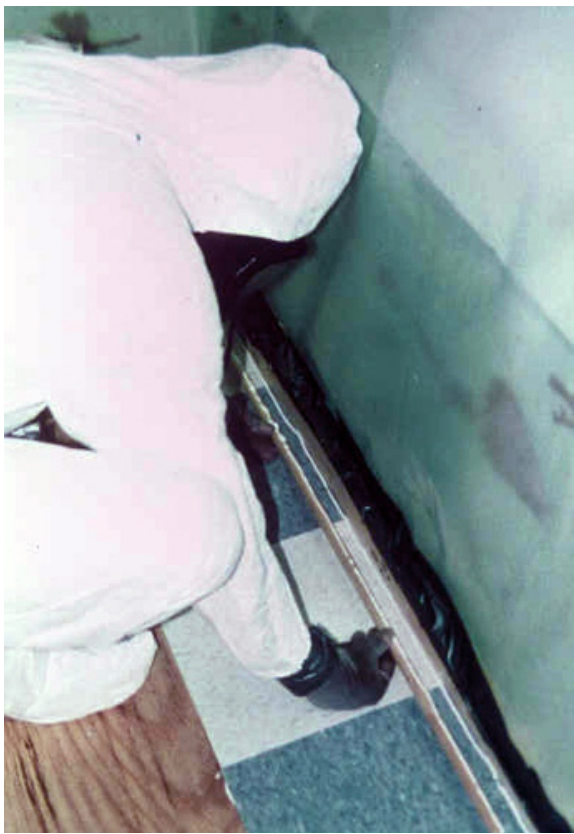
FIGURE 13.1 Encapsulating a floor with vinyl tiles
