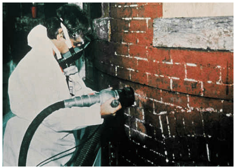
FIGURE 12.18 Vacuum blasting is not often used on housing.
