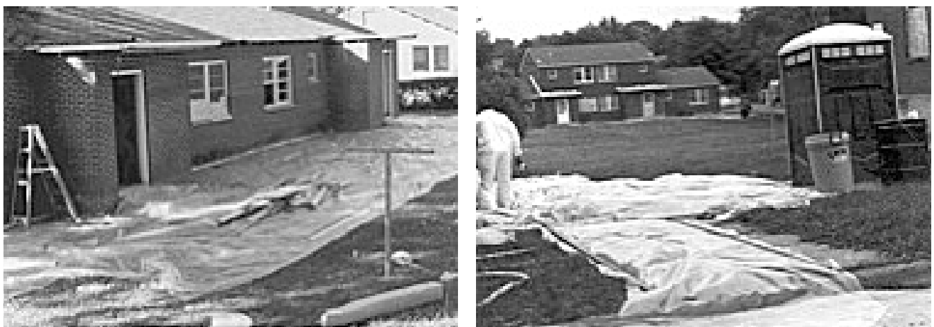
FIGURE 12.8 Line surfaces with plastic in the work area (left) and pathways (right)
