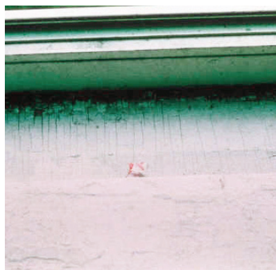
FIGURE 5.4b Alligatoring paint
