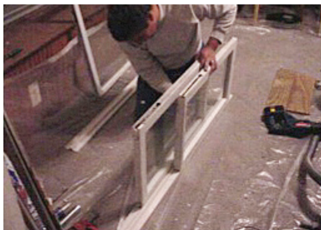
Figure 11.13 Fit sashes into jamb liners.
