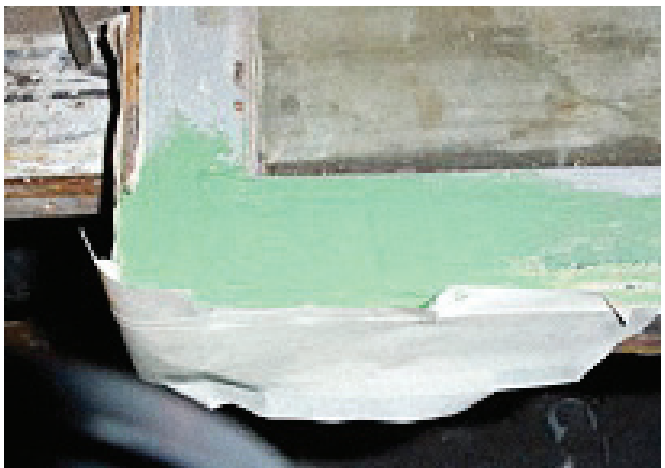
FIGURE 11.10 Rebuild damaged sash with filler or putty.
