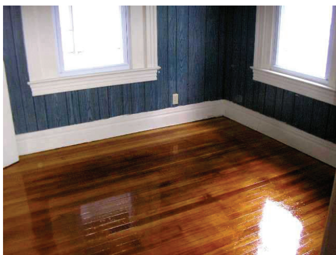
FIGURE 15.6 A floor that may be tested.
