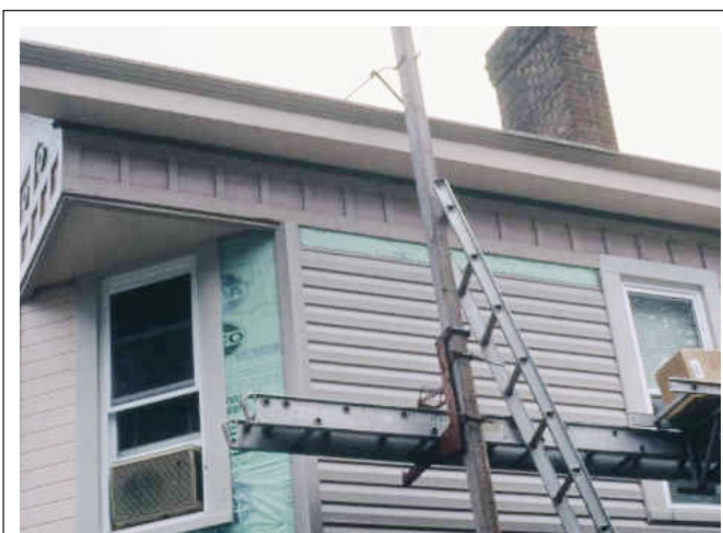
FIGURE 12.6 Installation of replacement siding.
