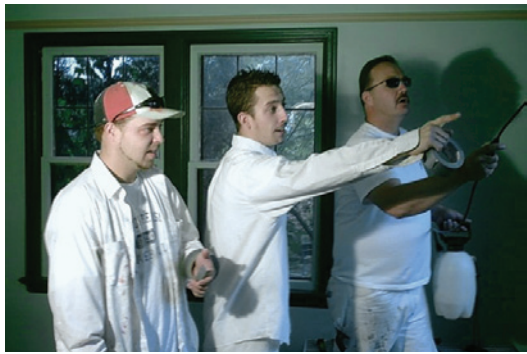
FIGURE 14.9 Inspecting for completeness of the work performed.
