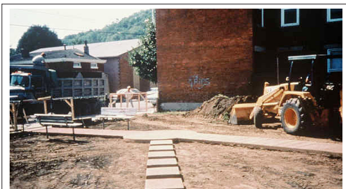
FIGURE 12.22 Replacing resident pathway after soil removal.
