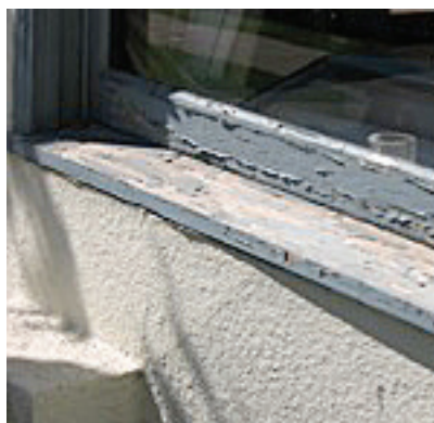
FIGURE 5.4a Peeling paint
