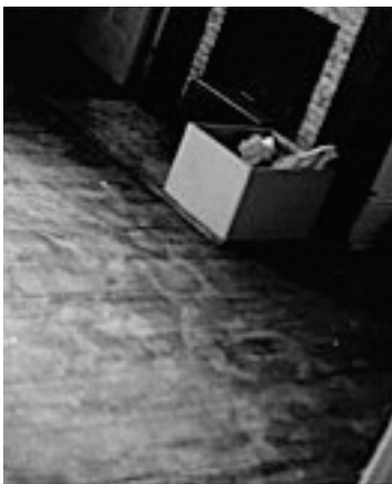
FIGURE 15.3 Visible Dust Indicates Recleaning is Needed
