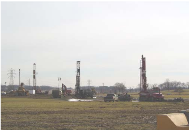
Figure 2. Multiple drill rigs at underground coal mine fire.
