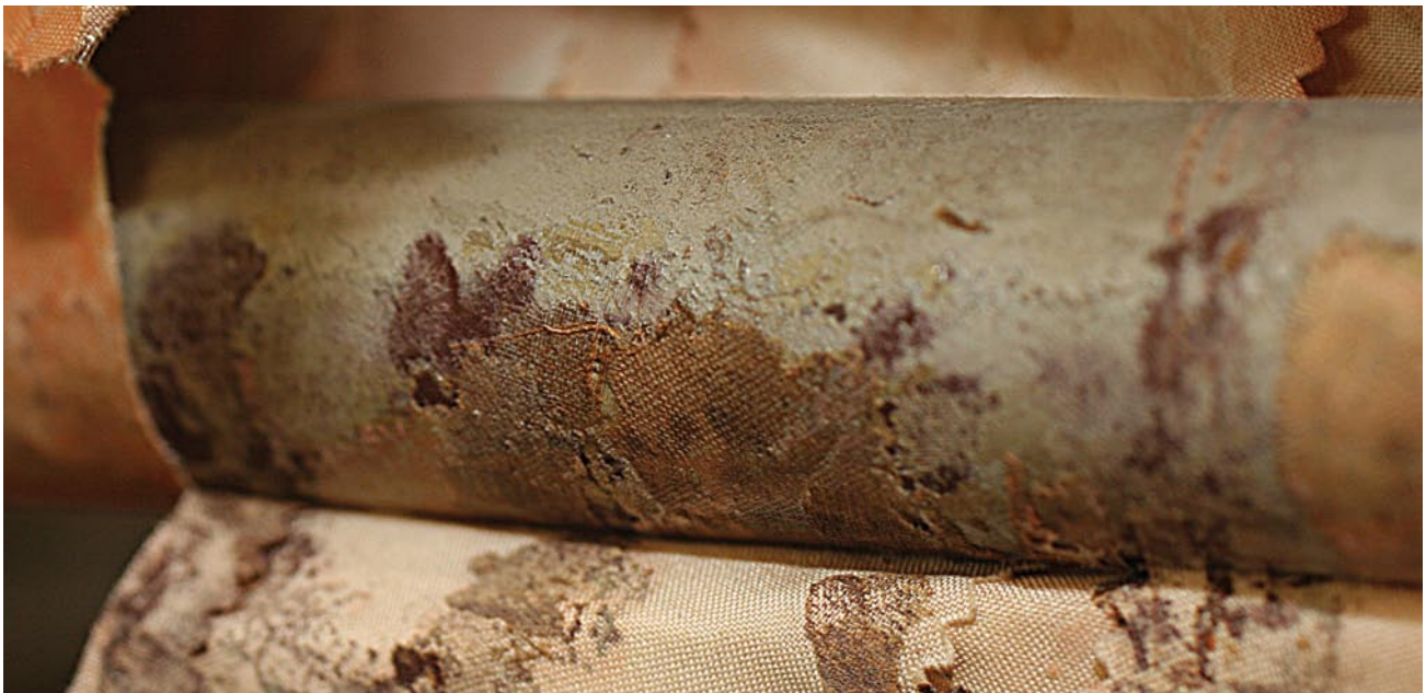
Figure 6-15. Rust on structural components.
