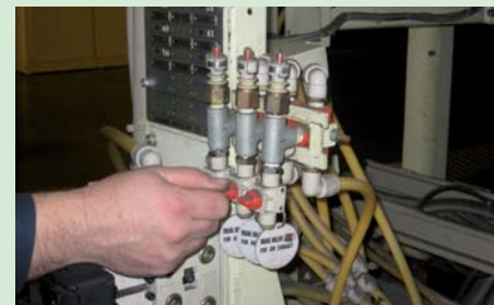
Bleeding air pressure by opening a valve
