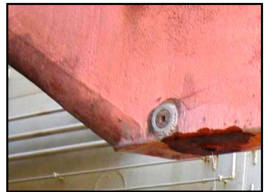
Figure 3. A vent plug indicating leaking product.
