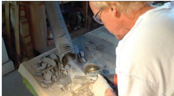
While grinding stone, a worker uses local exhaust ventilation to remove silica dust and reduce his exposure.
