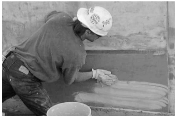
FIGURE 7. Sack and Patch Concrete: Sacking is a finishing process for fine cement surfaces, to fill small pin holes and other imperfections. It involves applying a wet cementitious slurry with a rag, followed by application of very fine, dry, usually 100% silica sand using a handheld burlap sack material. It is often done in conjunction with other patching tasks, although it was sampled in this study only when done separately from other types of patching tasks.
