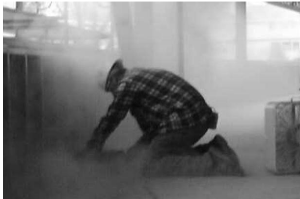
FIGURE 6. Surface Grinding: Rough walls, floors, and support columns were leveled using the flat surface of a 4.5 or 7 inch diameter surface grinder with an abrasive or diamond disk. At times this process takes an entire shift, while many times it was employed for only a small area or intermixed with patching.
