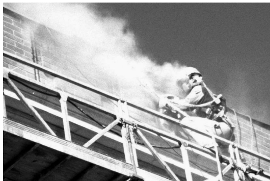
FIGURE 5. Tuck-Point Grinding: During masonry wall renovation, tuck-point grinding removes old mortar from between bricks, using a right-angle grinder. Usually, grinding occurs for half a shift and “tuck pointing” e.g. replacement of mortar, occurs for the remainder of the shift.
