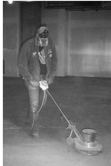
FIGURE 8. Floor Sanding: Floor sanding is a finishing process for smoothing cementitious floor underlayment products. The floor sander was a 16 inch diameter sandpaper disk and is operated from a standing position. This process was interrupted frequently to move obstructions out of the way.
